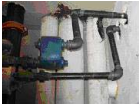
Steam Lines Installed For New HVAC
