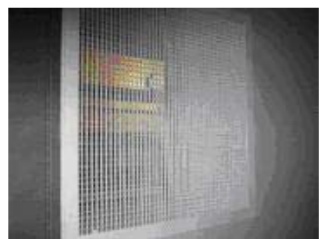
Grill Has Been Installed In Stairway
