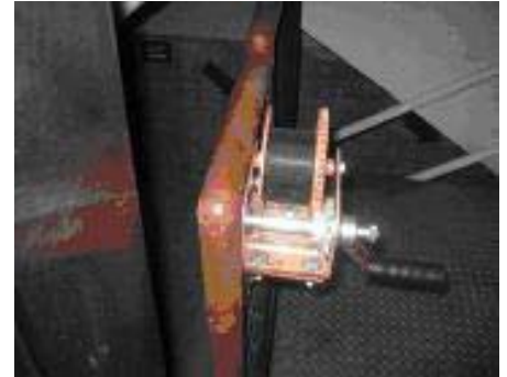
Overall View From The Elevator Car
