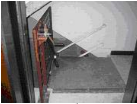
Side View Of The 4 th Floor Platform
