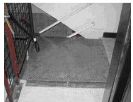
4 th Floor Platform From Elevator Car
